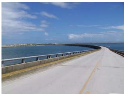
Bonner Bridge Summer 2013
