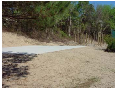
This is the site of the soon to be completed gazebo and basketball area at the park in Chichahauk.
