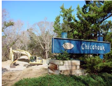
Work was well underway in mid-January on the Chicahawk Bridge.
